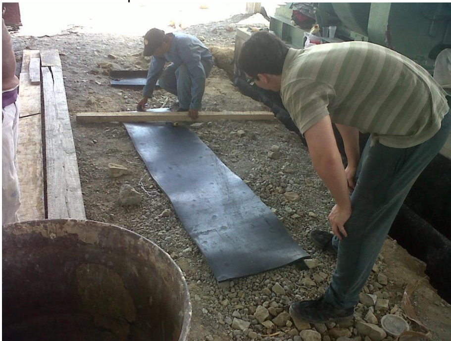
Annex #18 Author with finished antisismic rubber installation job.
